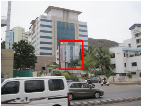
Onio's building and close-up view of existing banner.
